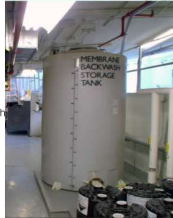
Treated Effluent in storage tanks in Basement
