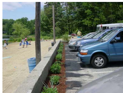
This parking lot buffer in Littleton captures and infiltrates stormwater runoff.
