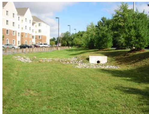
This infiltration basin collects and infiltrates runoff from the adjacent parking area.
